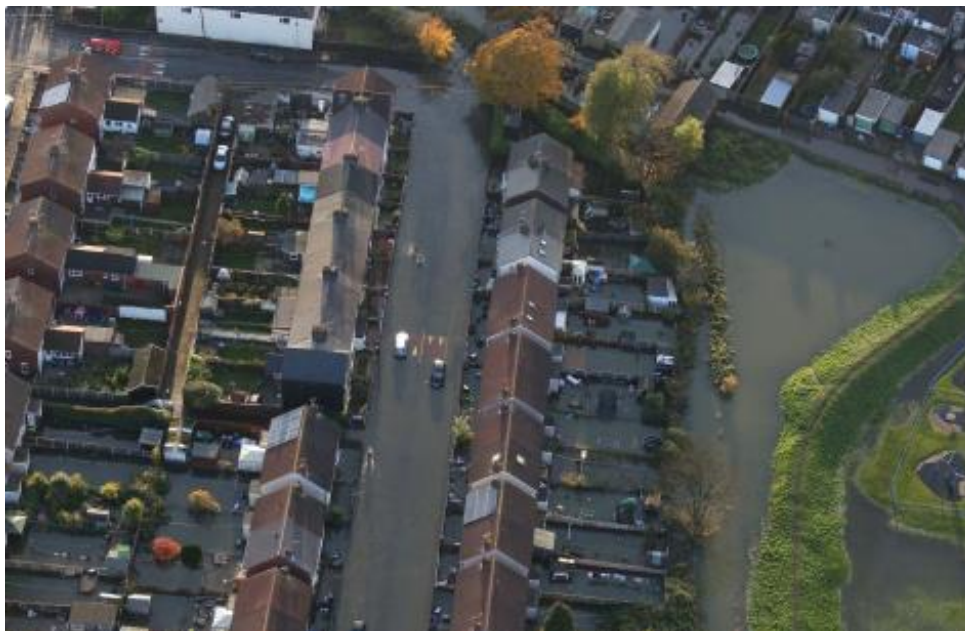
Figure 8. Flooding at Bentley during the 2019 flood event.
